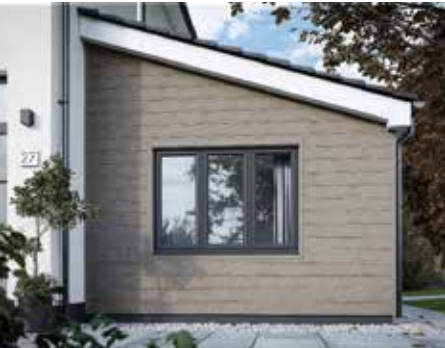
Horizontal Cement Boards
